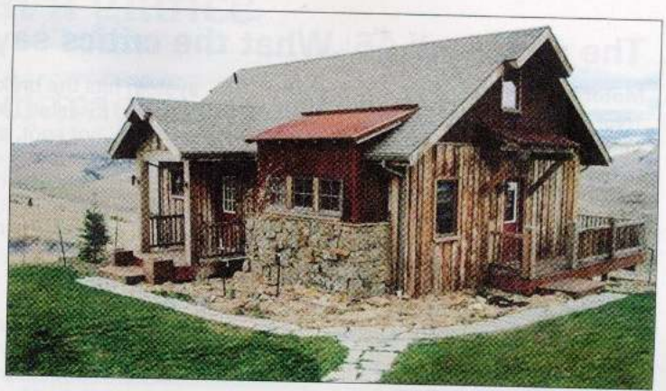
5 ▲ Livingston, Mont. This 1,100-square-foot cabin is located on 25 fenced-in acres abutting state land. The home is fully furnished and features two native-rock fireplaces and a wraparound porch with panoramic views. The home is off the grid, utilizing both solar panels and wind generators. $360,000. Mary Ackermann, ecoREsource Properties, (406) 587-2950
